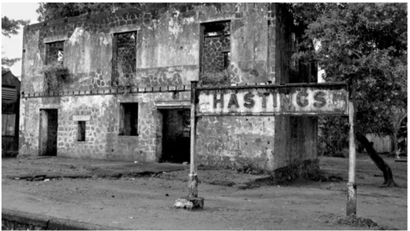
Noncreative destruction: abandoned Hasting railway station on the way to Bo in Sierra Leone © Matt Stephenson:
